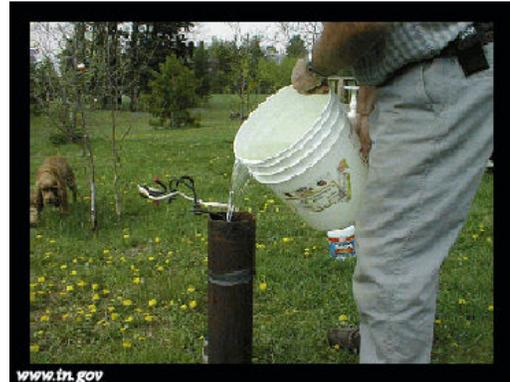
**Step 5.** For wells connected to a plumbing system, open all inside and outside faucets and pump water until you notice a strong odor of chlorine at each faucet. If you do not smell chlorine after running all faucets for 15 minutes, increase the amount of chlorine by one-half of the original amount used and repeat the procedures.
